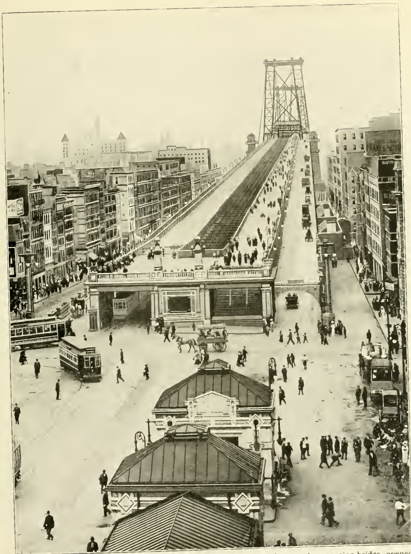
WILLIAMSBURG BRIDGE APPROACH—A combined cantilever and suspension bridge, opened Dec. 19, 1903, crossing the East River from Delancey Street, New York City to Broadway, Brooklyn. Total length 7200 feet, width 118 feet, height 135 feet clear. Cost, $10,000,000.
